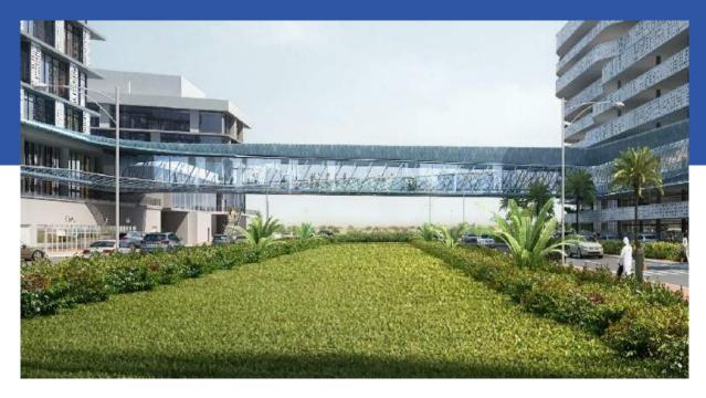
The Pedestrian Link Bridge is located in Nad Al Shiba First Community in Dubai. The proposed structure will connect the under-construction Emirates NBD Parking Building on Plot no. 6184109 & the existing Emirates NBD Offices Building on Plots no. 6184115. The bridge main structural elements are steel structure box shape truss spanning between two building i.e. parking building & podium building.
